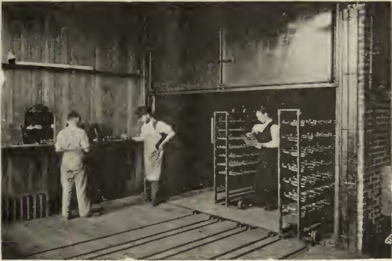
Drying Ovens, Japanning Dept.—Edison Phonograph Works.
